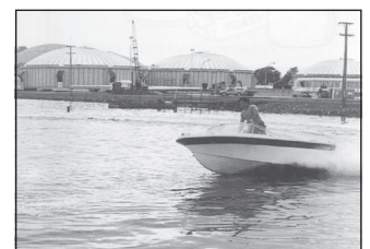
Figure 1.19 Oxidation pond being stirred up by a boat in order to increase the oxygen in the water
